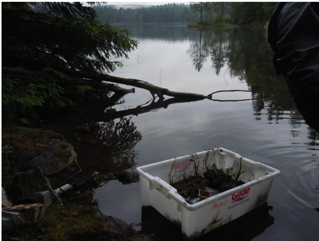
Photo 1. Breisjøen, location 1, with the maximum water level. Start of work. Attempts were made to dig individual plants into biodegradable paper pots. 19.07.2019.
