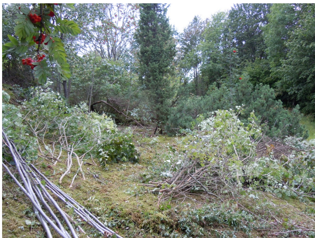
Photo 4. Clearing of the bushy slope. 6.09.2019.
