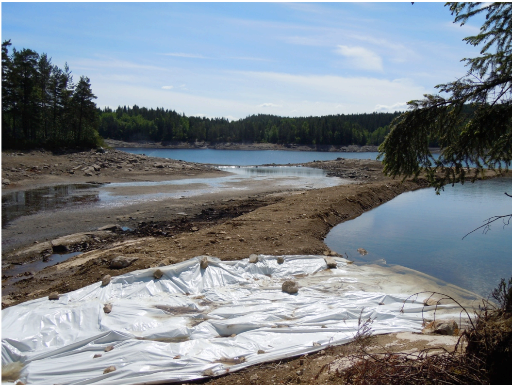
Photo 4. No 2 (blue) Dam (on right), “our dam” no 3 and wet area no 3+ (center), No 4 (red) Irrigation (left) in the northern part of the lake.
