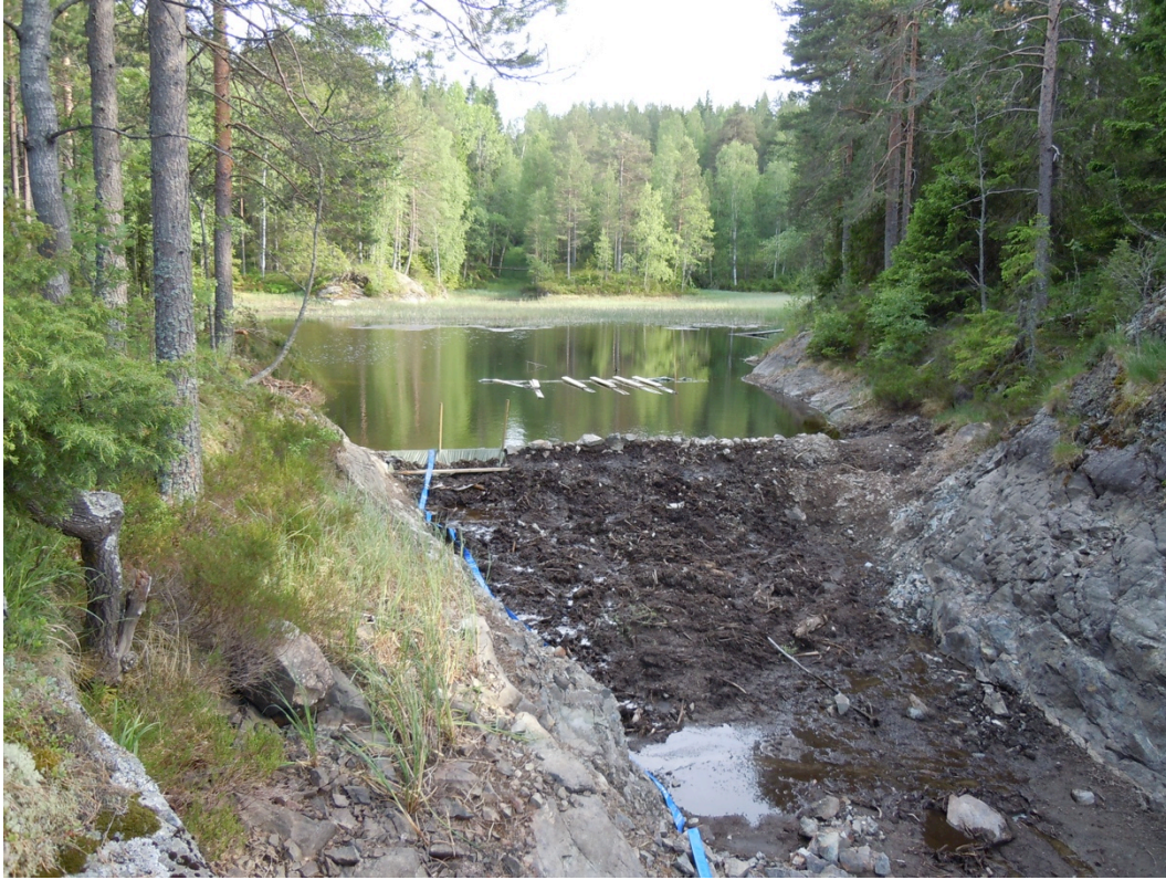
Photo 3. No 1 (blue) Dam in the southern part of the lake.
