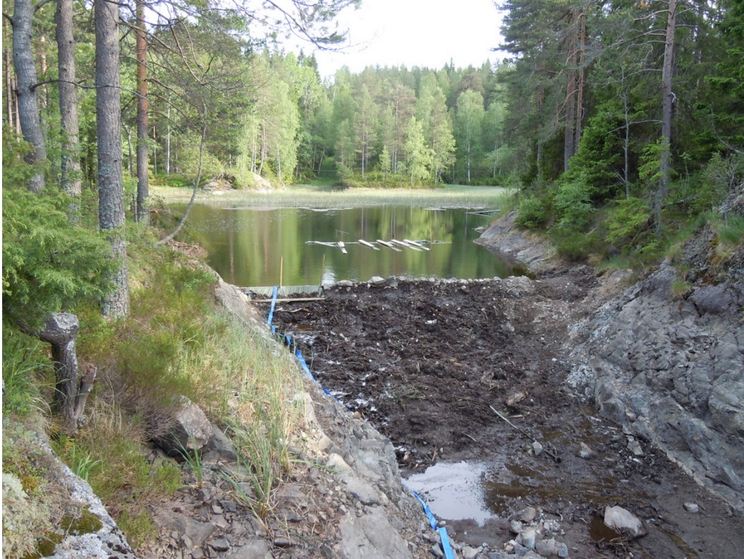
Photo 5. No 1 (blue) Dam in the southern part of the lake. 11.06.2020.
